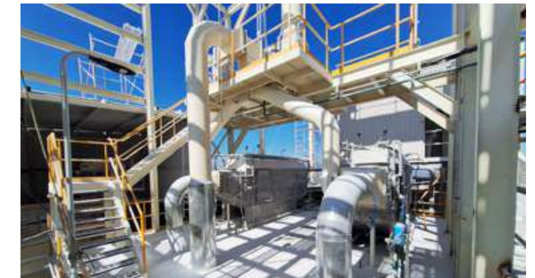
Evaporated Water Recuperator in the Hydration Process – Progreso Plant
