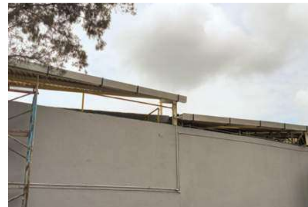
Roof gutters to recover rainwater at the Progreso Plant
